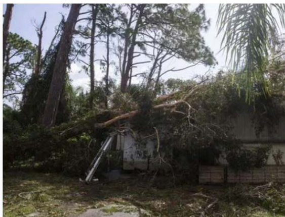
Wind and flood damage to a home in Bonita Springs after Hurricane Irma. Damage not fixed by Jan. 1 can lead to a reduction in property valuations that could save money for affected homeowners. (Photo: Nicole Raucheisen/USA Today Network-Florida)
